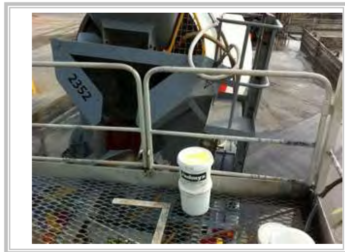
Figure 2: The adding of Radmyx at the batch plant
